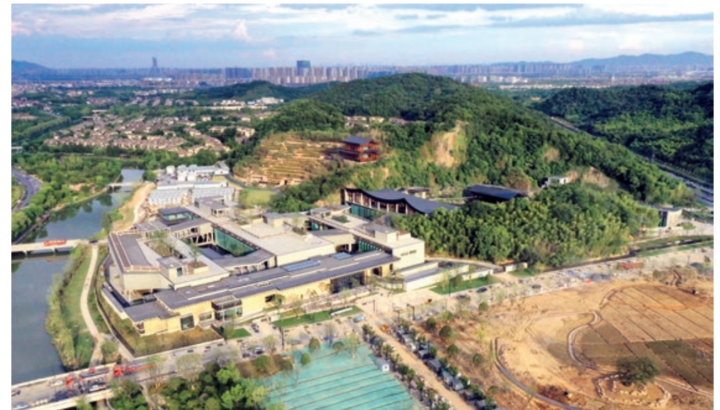
The National Archives of Publications and Culture in Hangzhou © Amateur Architecture Studio
